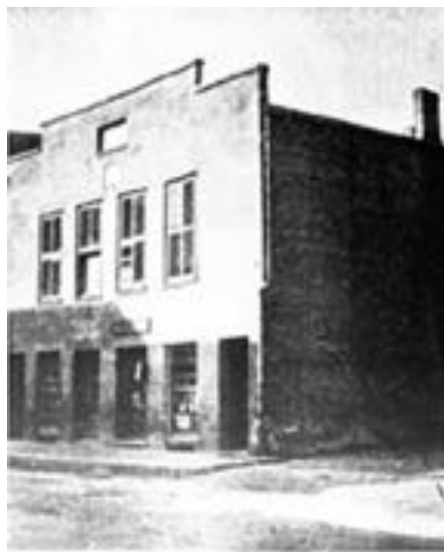
Sanford Street Church, c. 1911
