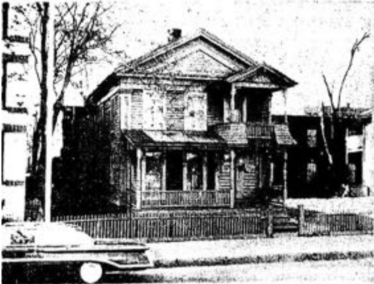
Abolitionist John Brown's home at 31 Franklin St., now occupied by Mr. and Mrs. William F. Brewster, will be demolished soon by the Springfield Redevelopment Authority. Brown is said to have lived here between 1845 and 1849 while he was in the wool business.
