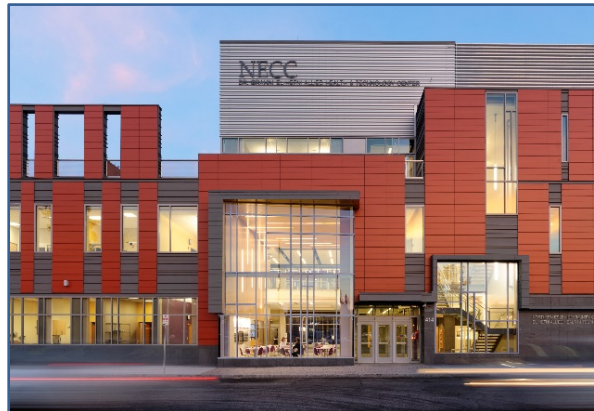
NORTHERN ESSEX COMMUNITY COLLEGE LEED-SILVER CERTIFIED
