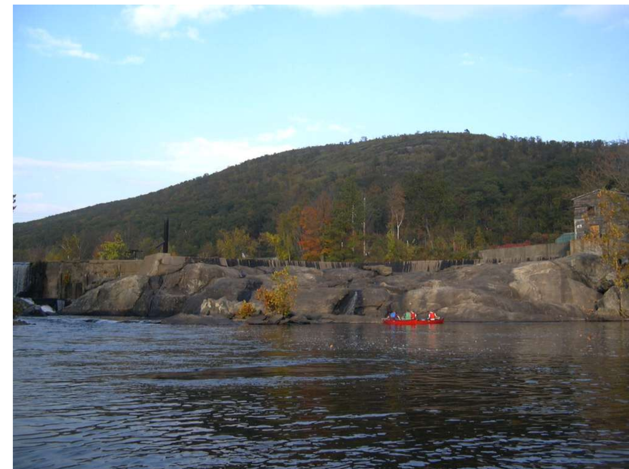
Figure 2: The dam forming Russell Reservoir (Station 30).
