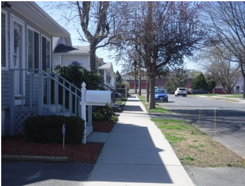
Location: Windsor Street Description: Sidewalk- both sides of street (but not continuous – see picture 3 and 4); houses close to street-obstruct vehicles from seeing pedestrians; sidewalk and road service excellent; grass strip acts as barrier between sidewalk and road.
