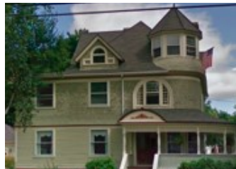
69 Western Avenue - Lewis Allen's home and site of his murder.
