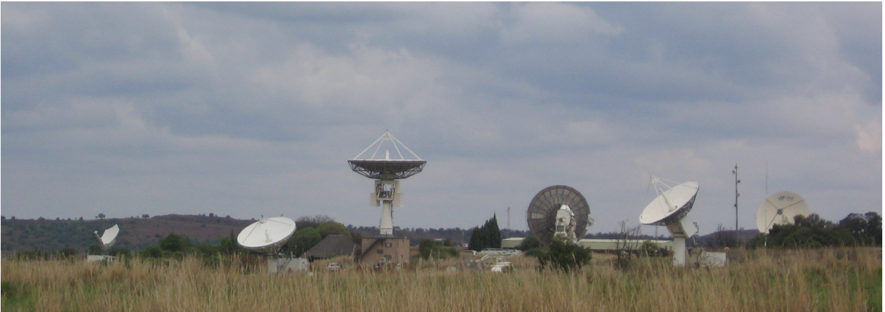
Illustration 4: The CSIR Satellite Applications Center at Hartebeeshoek near Johannesburg. Special antennae track satellites as they pass overhead and download images using radio waves.
