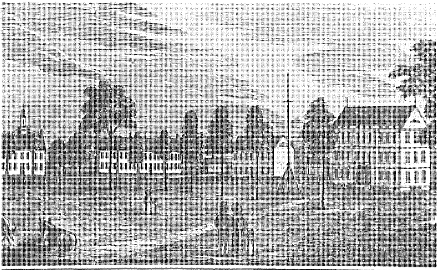
Western view of the Armory Buildings, Springfield.
