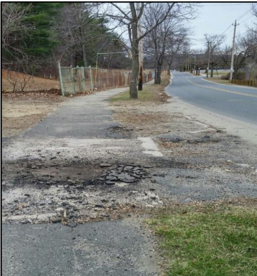
Figure 7: A severely torn up sidewalk along King Street
