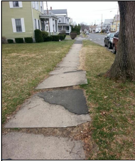
Figure 6: A highly cracked and unlevel sidewalk on Charles Street
