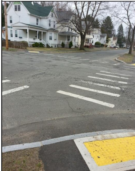
Figure 5: An intersection with well-painted crosswalks and pedestrian detection pads on the corner of Charles Street and Jefferson Street
